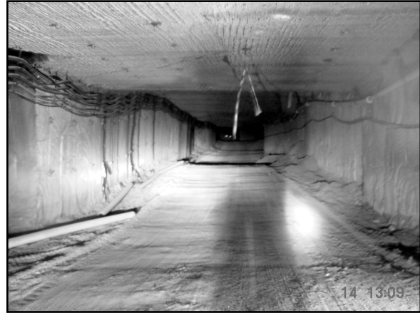
Underground salt road along which waste will be transported in a pipeline
